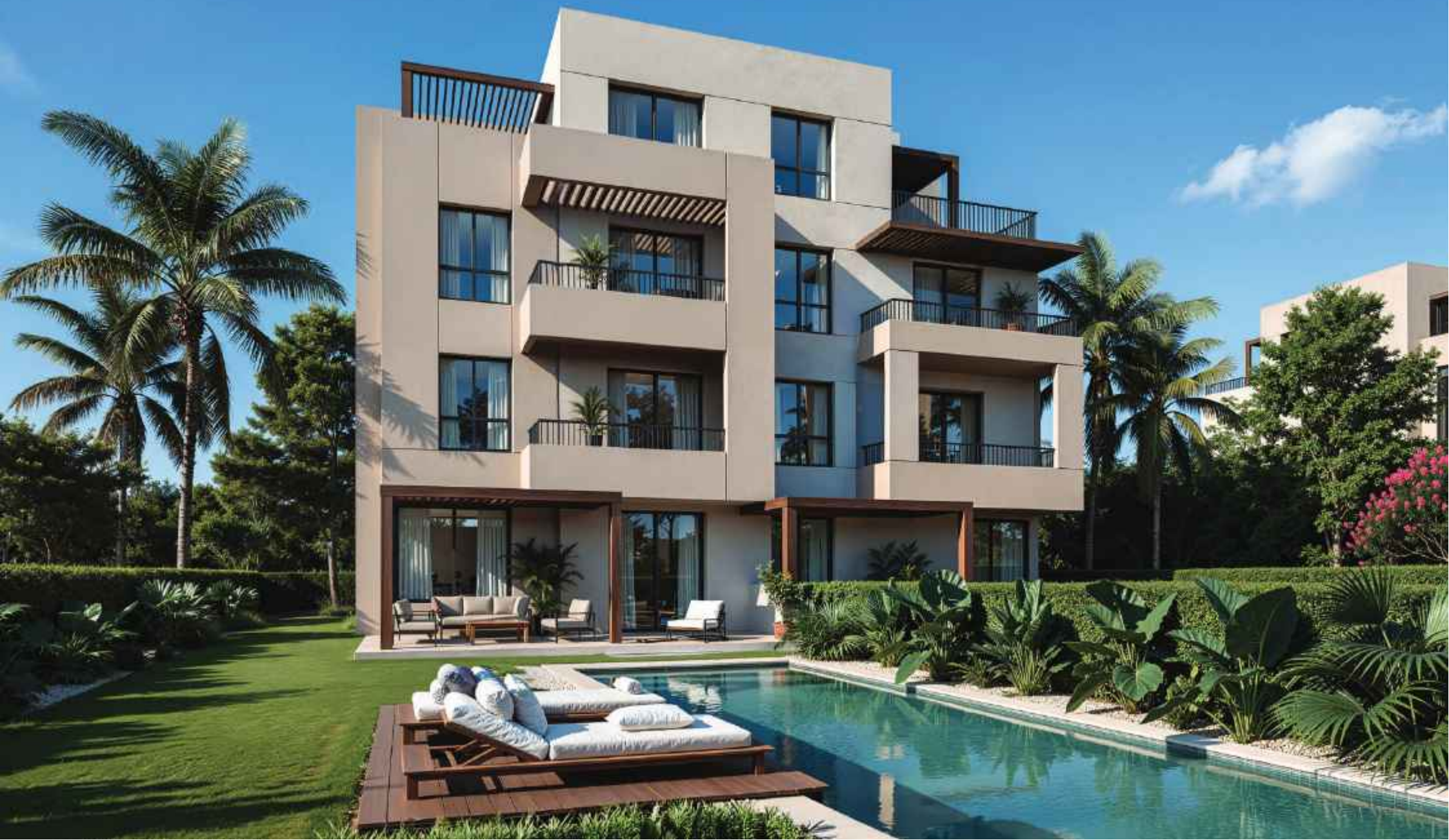
Parkside Residences A Back View
